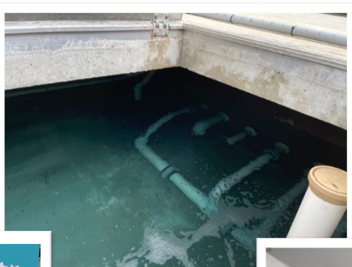
Installed secondary disinfection system and run system 24 hrs./day
