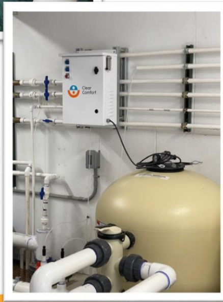
Installed secondary disinfection system and run system 24 hrs./day
