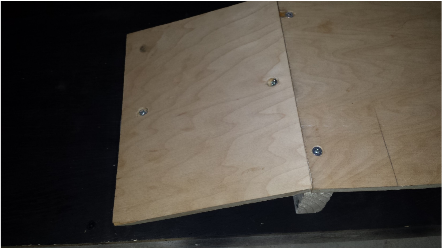
Figure 6 Ramp Incline Countersunk Screws Centered on Board
