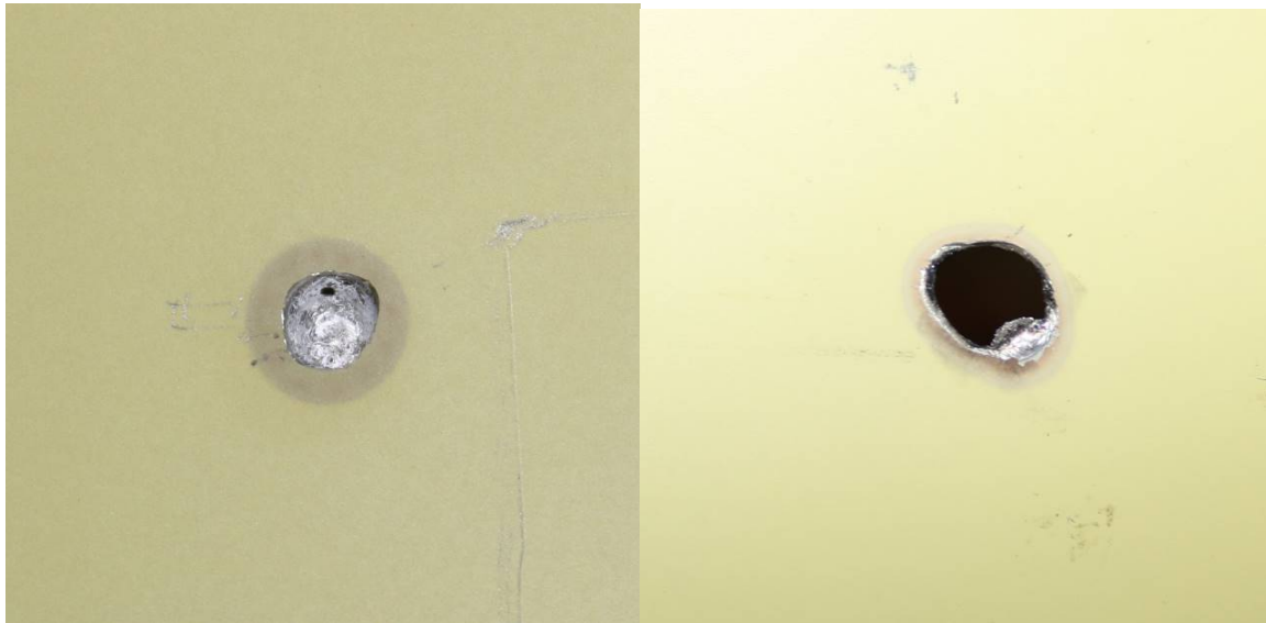
Figure 8: Left: Interior-side damage, and right: through hole
