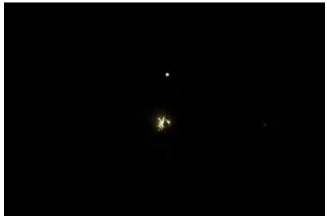
Figure 64: MN-1I11-2, during test, external sparks on J2 & J3
