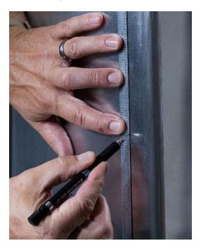
Step 3: Obtain JAM Trip tape of desired trip thickness and remove enough backing material to start work with the tape. Note on roll of tape, there is a starter tab. Apply the tape by hand following marked line.
