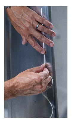
Step 4 (if necessary): If the line of trips is longer than the standard package length, cut the end of the tape with sharp scissors or sharp knife just PAST the last dot before application.
