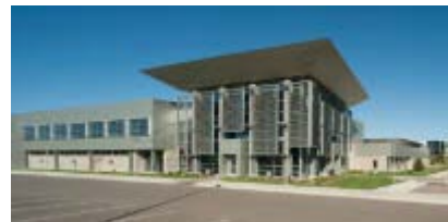
Figure 2. National Center for Aviation Training (NCAT)
